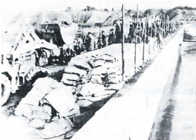
Reinforcing embankments of the Liujia Gorge Reservoir on the upper reaches of the Huanghe River before the advent of the flood peak.
