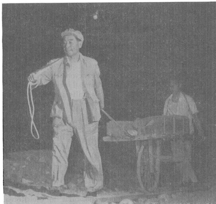
Chou En-lai hauling a cart on the night shift at the Ming Tombs Reservoir construction site
