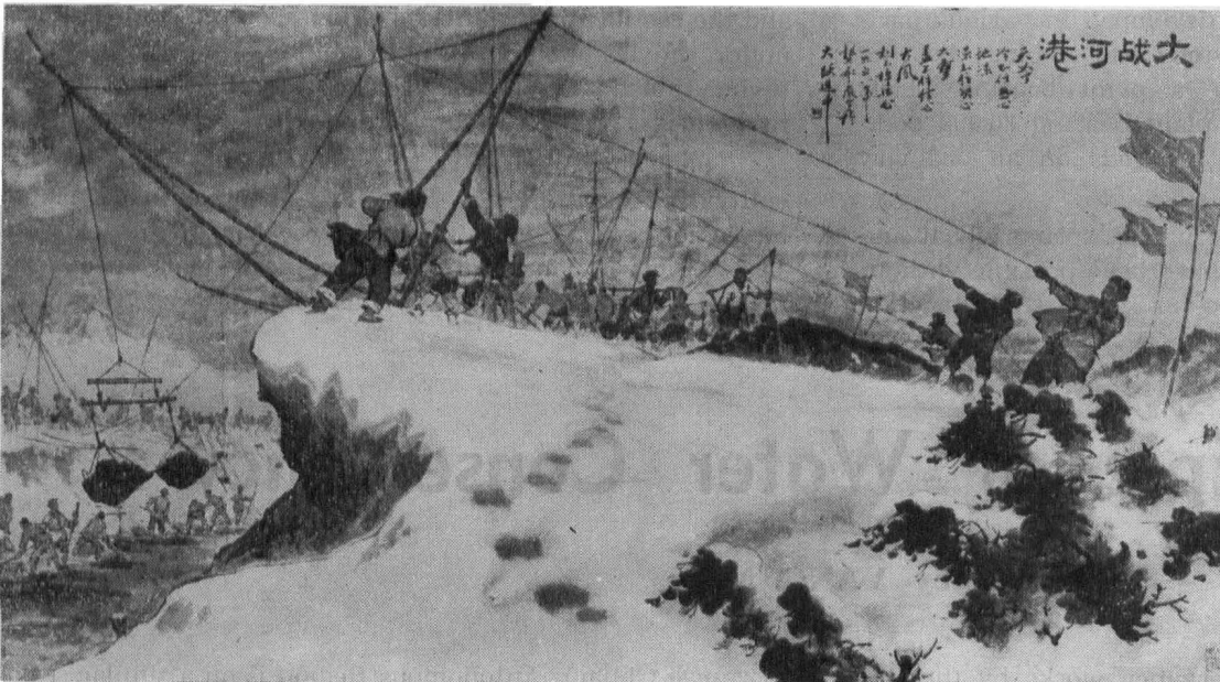
Dredging the canal
