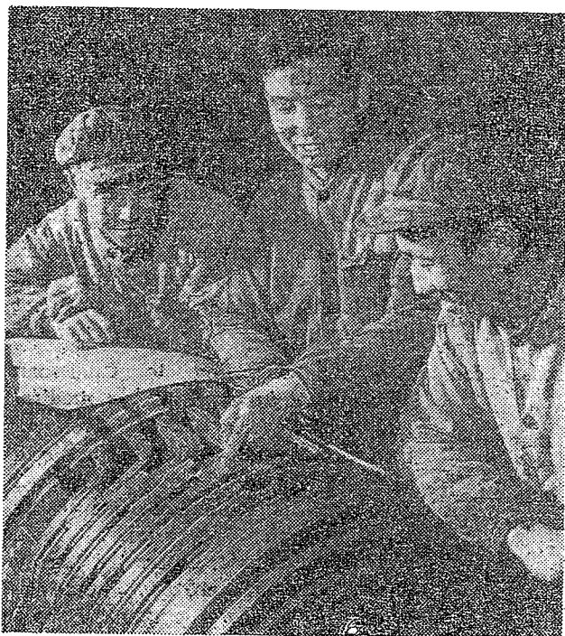
Workers and a technician at the Shihchia-chuang Heat and Power Plant studying how to better lower the temperature of a generator's rotor and increase power output.
