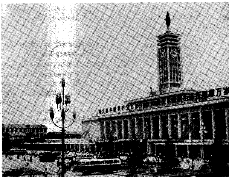
The new railway station in Changsha.
