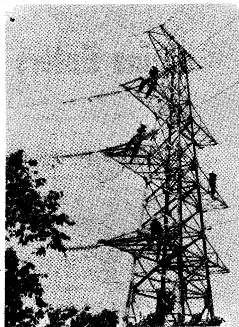
Putting up high-voltage wires in Honan Province.
