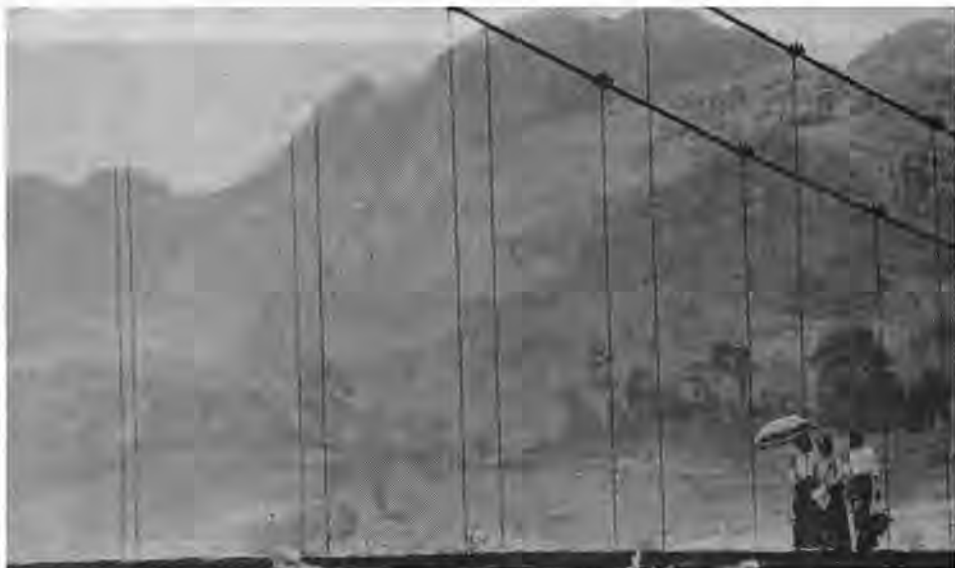
A cable suspension bridge across the Luosuo River.
