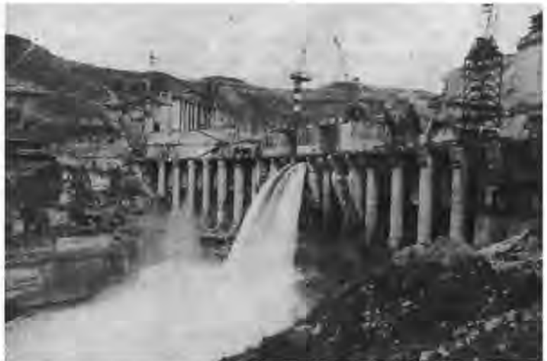
The Baishan hydropower station in Jilin Province now under construction. With a total installed capacity of 1.5 million kw, the station will ease the electricity shortage in northeast China's three provinces.
