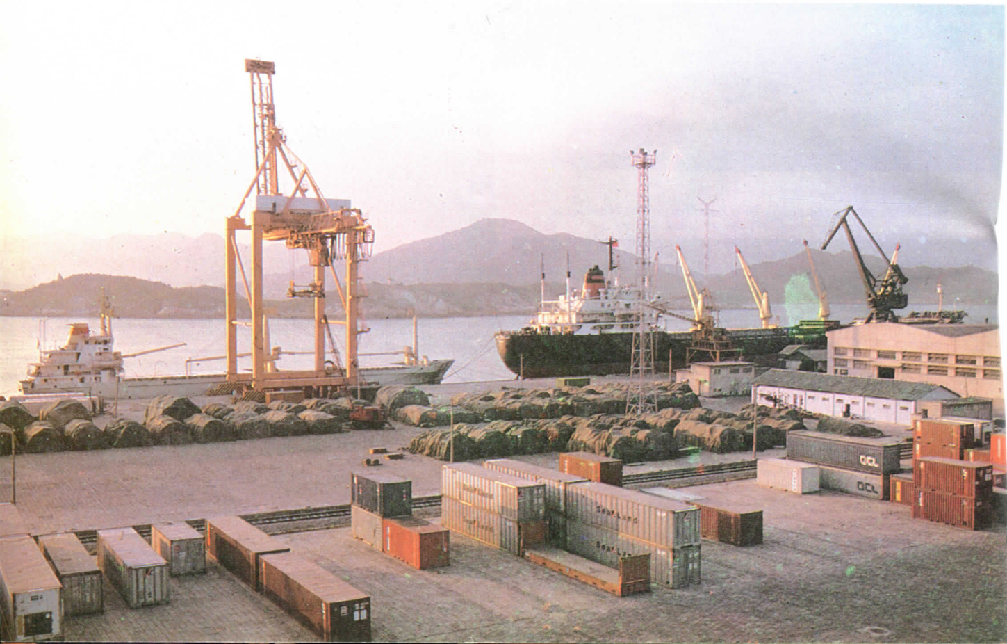
The new Dongdu Wharf for 50,000-ton-class ships.
