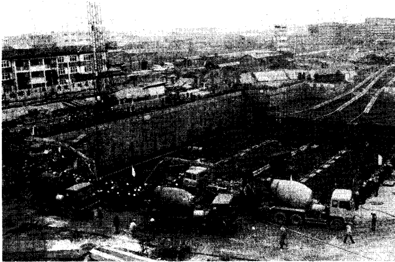
A Sino-British joint glass works under construction.
