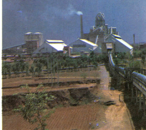
The Jidong Cement Works — the largest with an annual capacity of 1.5 million t
