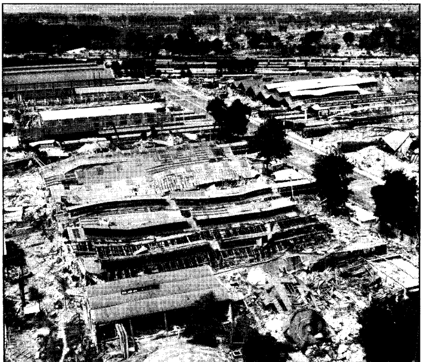
The Tangshan Locomotive and Rolling Stock Factory after the 1976 quake.
