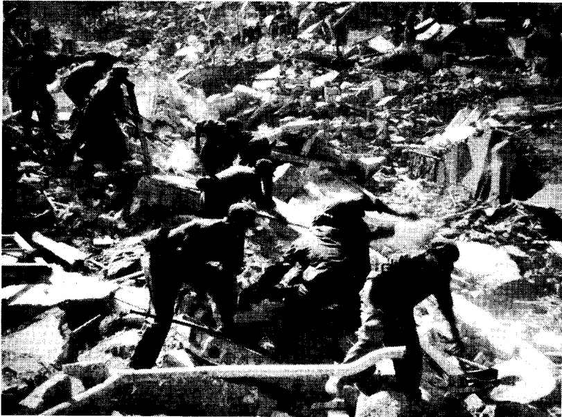
PLA soldiers working to rescue quake victims buried in rubble.
