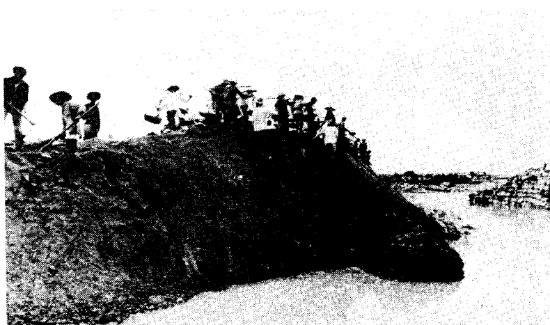
Farmers in Jieyang County, Guangdong Province repairing a dyke breached by the flood.
