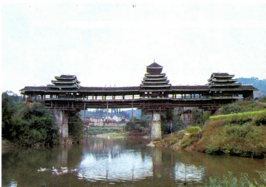
The Fengyu Bridge over the Xihe River.
