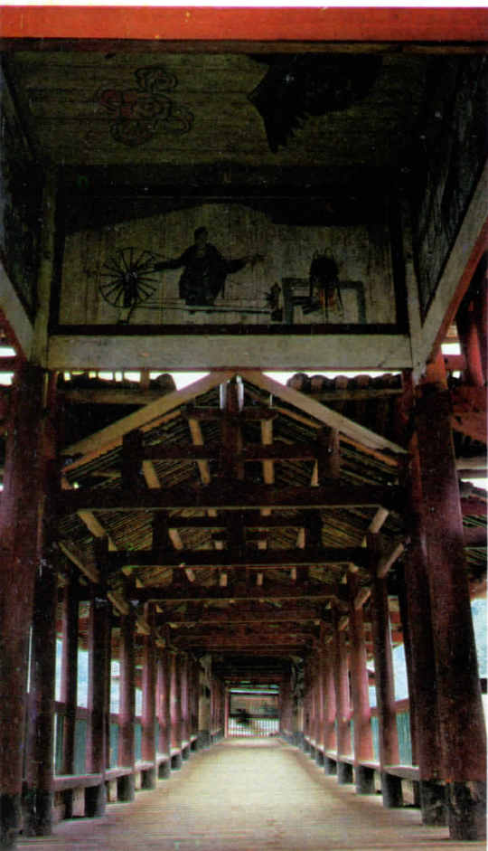
Inside the wooden Fengyu Bridge: meaning wind and rain, from which the bridge gives shelter.
