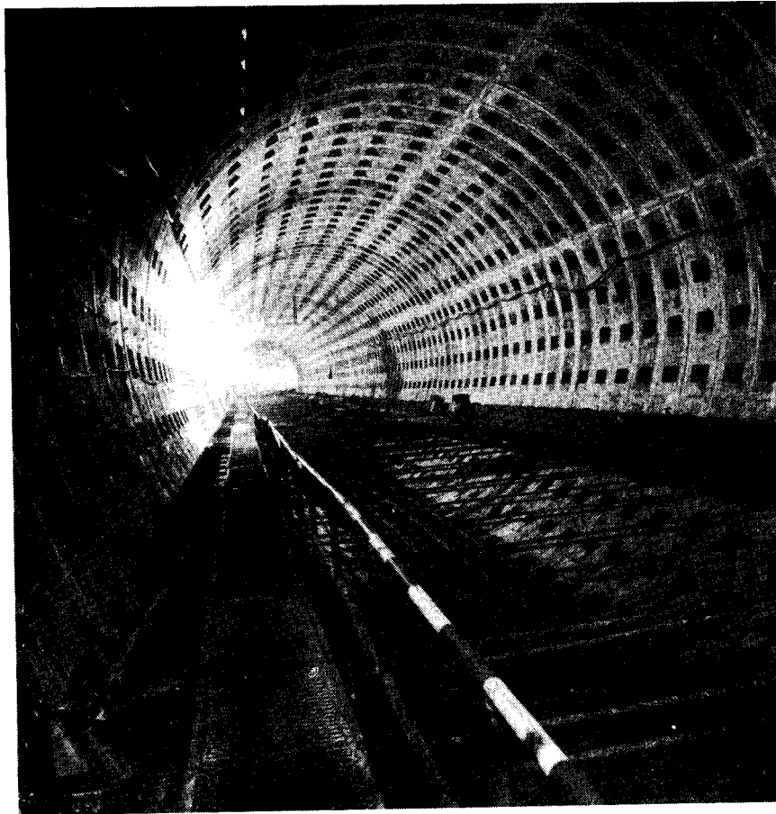
The second tunnel across the Huangpu River under construction
