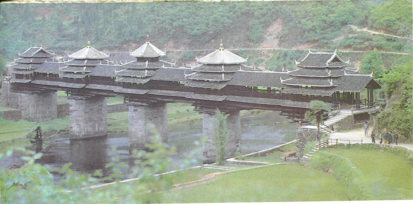
This typical Dong architectural-styled bridge is a key relic under state protection.
