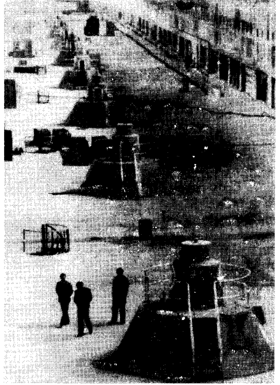
Water power: the final generating unit of the Gezhouba Power Station went into operation on December 10, 1988. HUA AI
