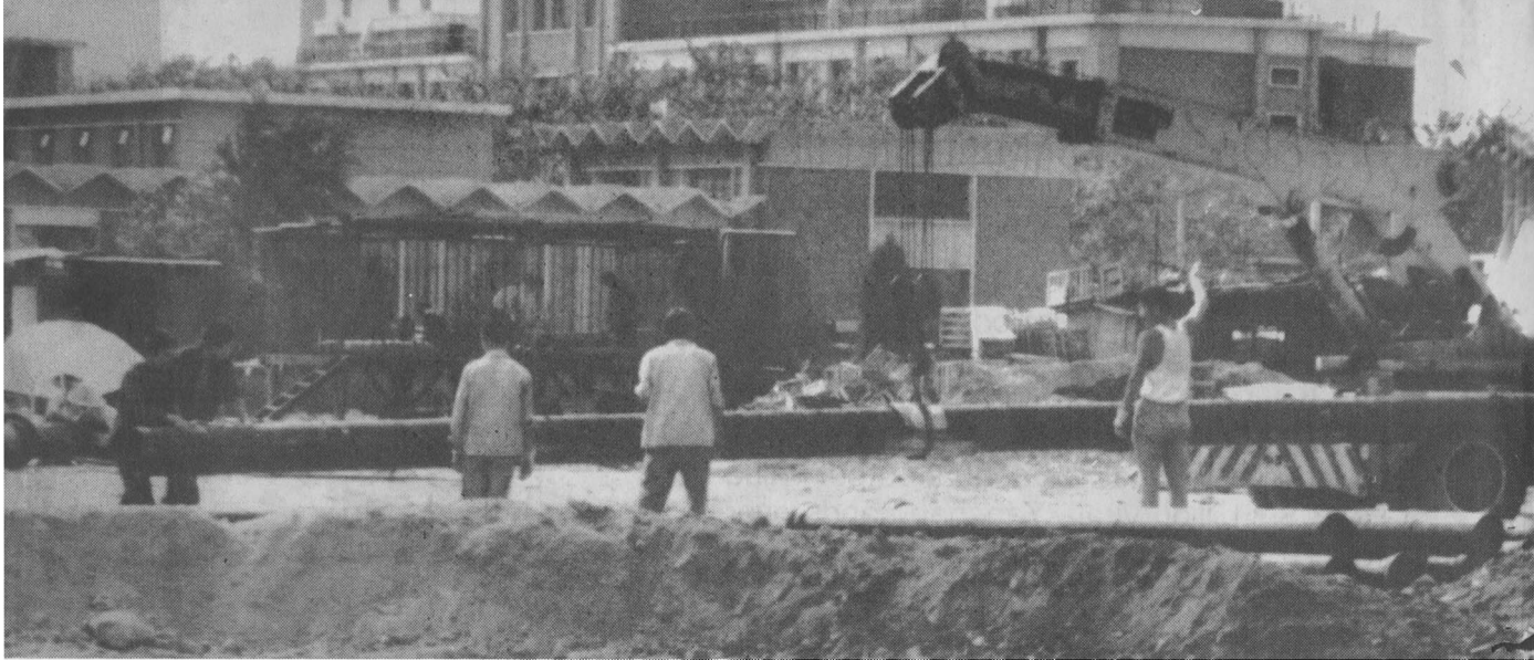
Workers laying underground pipes.
