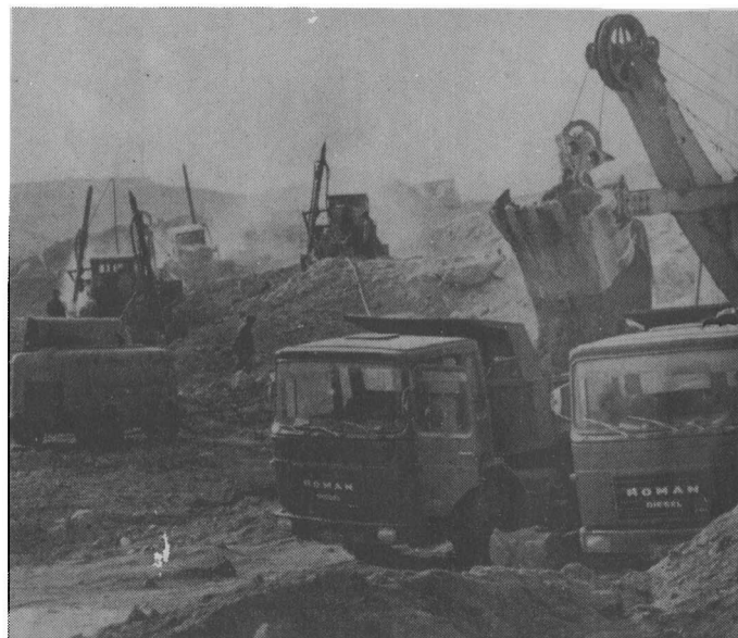
Earthwork in progress.
