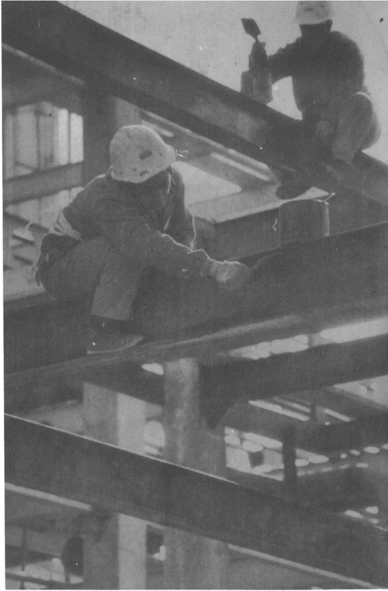
Painting overhead steel girders to prevent rust.
