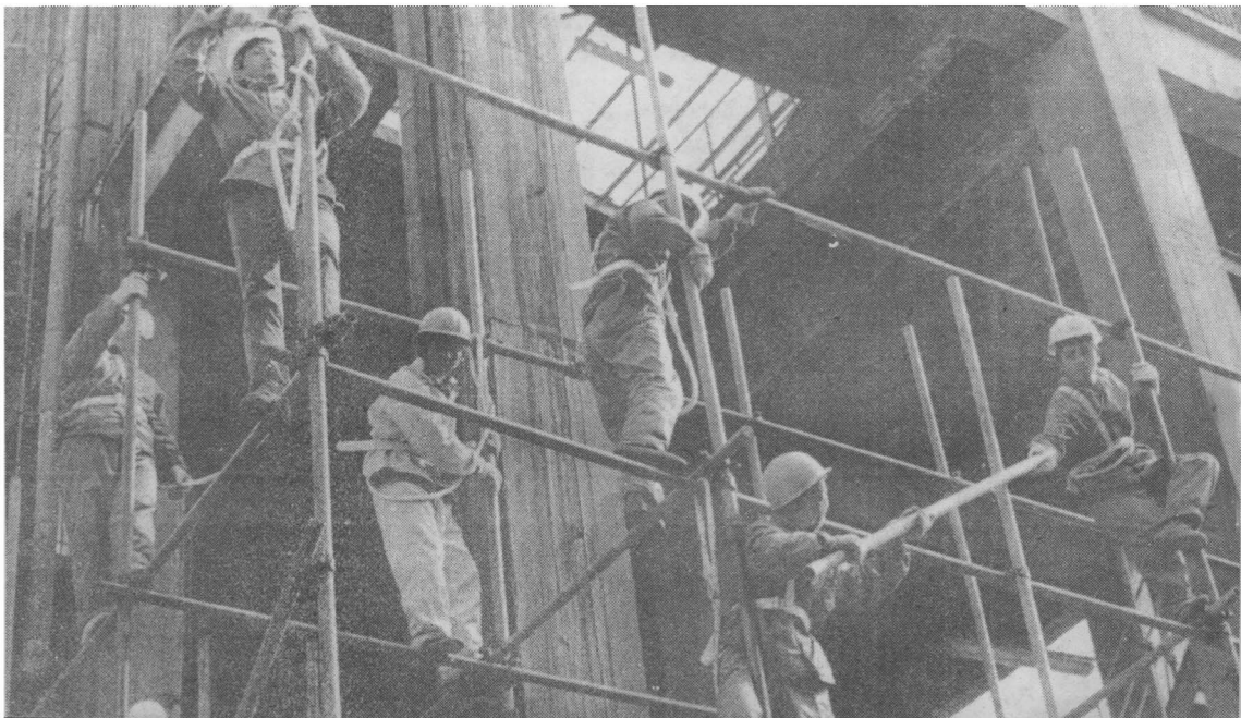
Scaffolders scaling the peaks.
