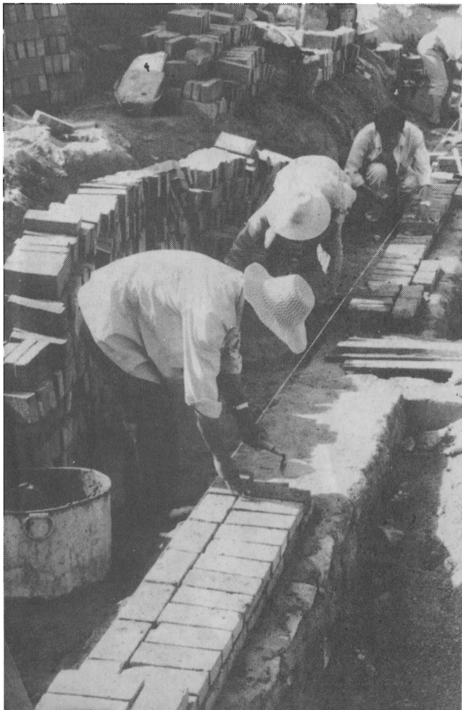
Workers putting up the factory.
