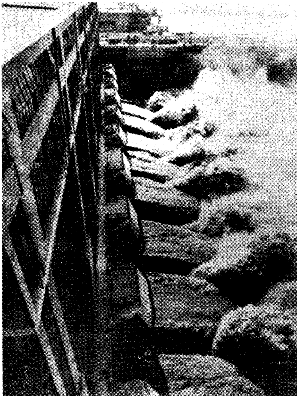
The 9-outlet sluice gate with a maximum flow rate of 20,000 cubic metres per second.
