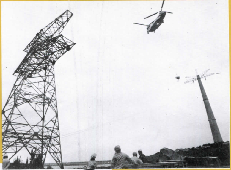
A helicopter is used to erect the power transmission line.
