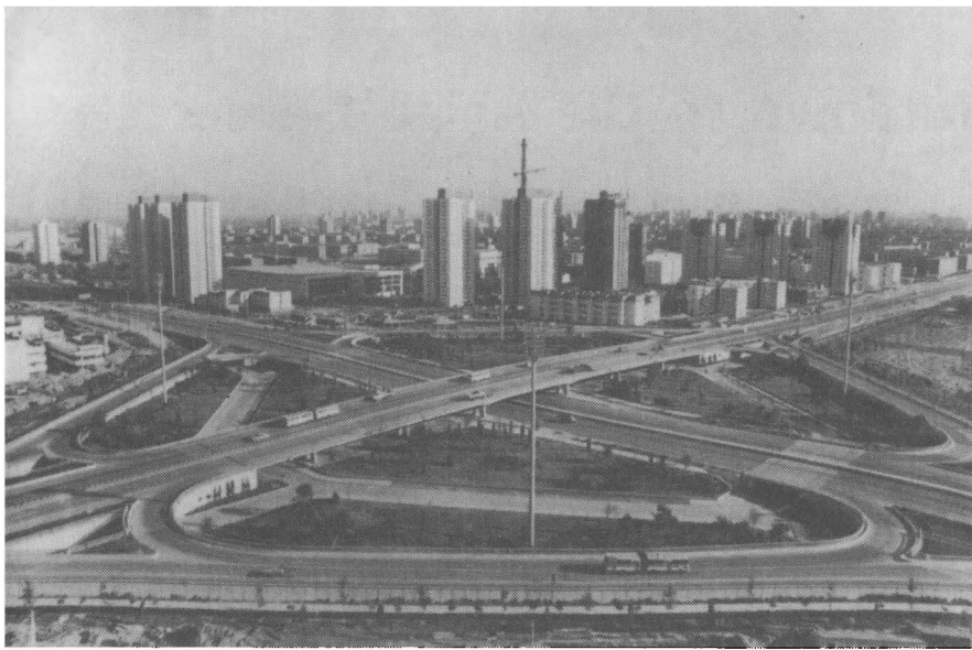
This newly built pass-over links all the stadiums and gymnasia with the Village of Asian Games.
