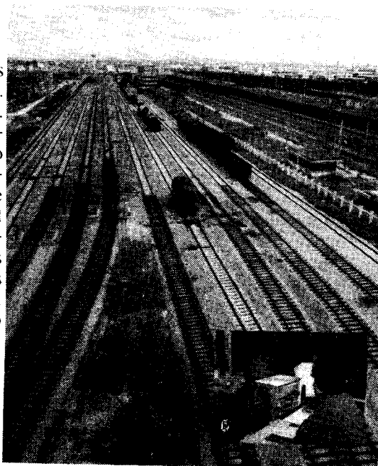
The Qinhuangdao Harbour Trainyard.
