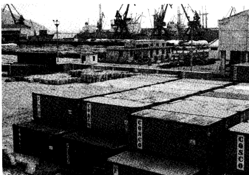
Container dock at Lianyungang Harbour.
