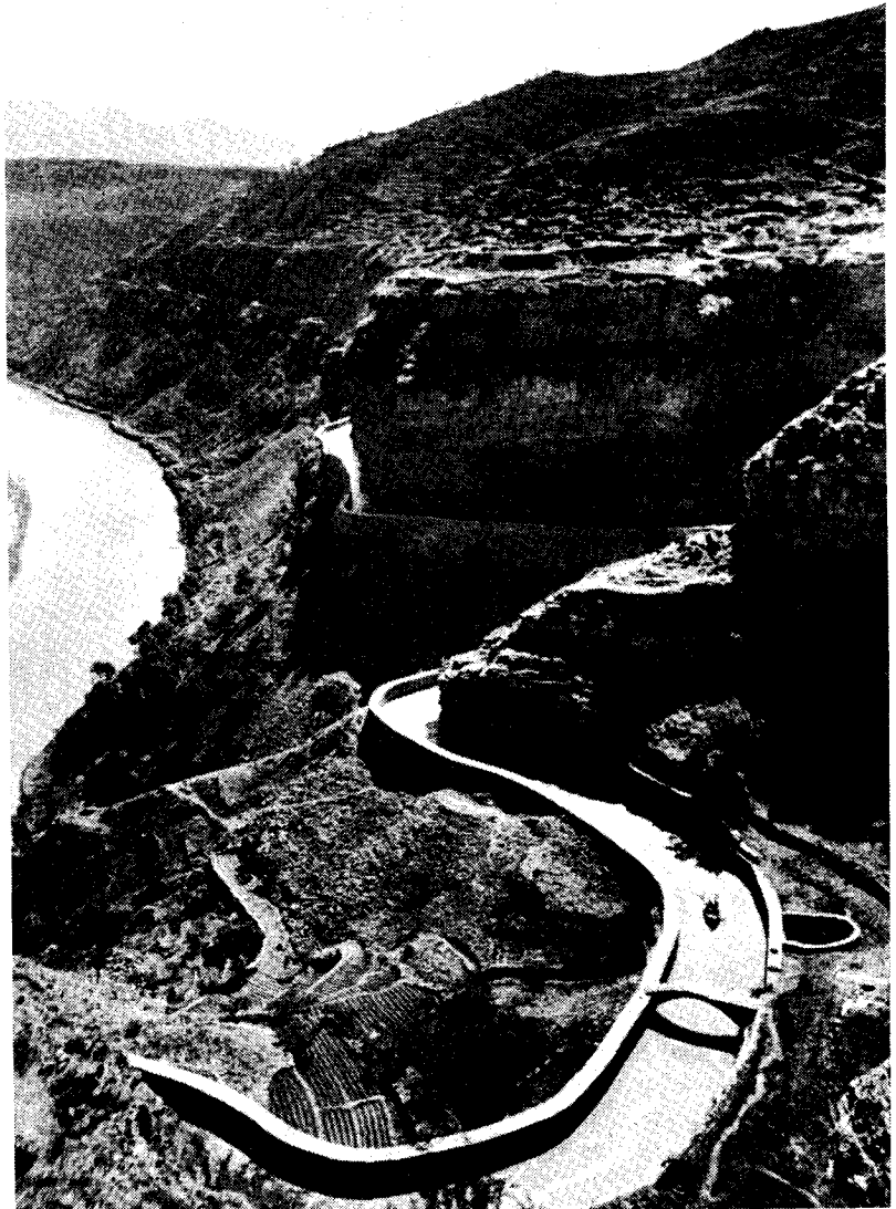
The Red Flag Canal, the 1,500-km-long irrigation ditch which farmers in Linxian County, Henan Province built over a ten-year period, provides water for crops even during dry spells in the mountainous area.
