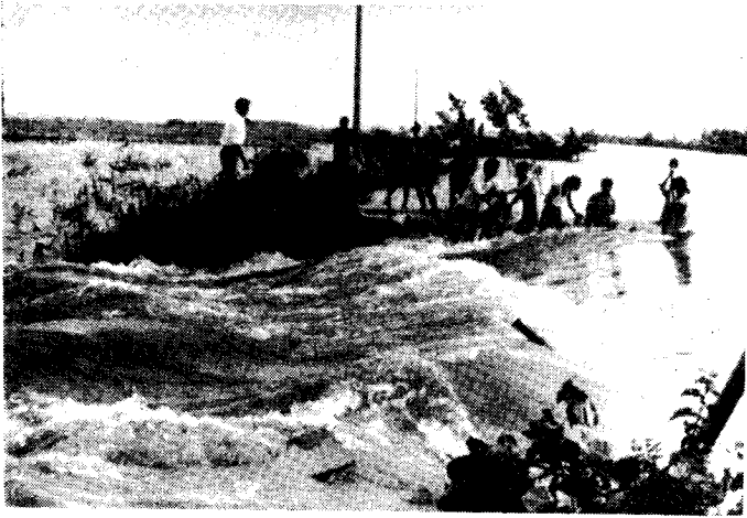
Soldiers and civilians strive to reinforce a dyke damaged by floodwaters.
