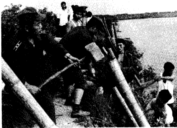
PLA men stationed in Suzhou City, Jiangsu Province, reinforce a river dyke.
