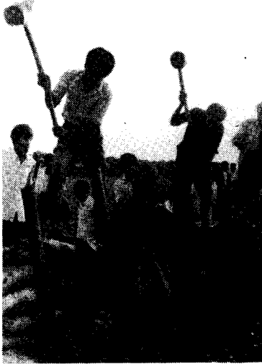
Farmers of Jianshou Township in Gaoyou City, Jiangsu Province, reinforce the river bank against rising water levels.
