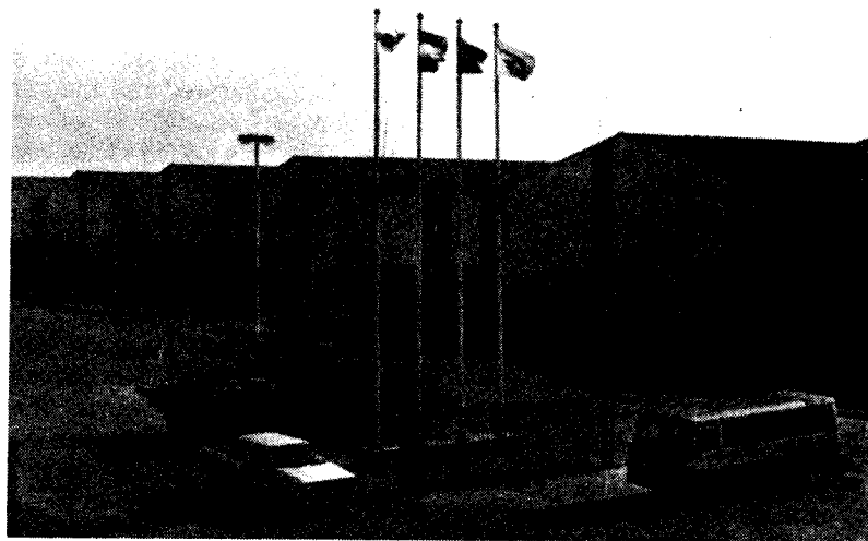
The bonded warehouse jointly set up by the Tianjin harbour and the Royal Nedlloyd Group N.V. Rotterdam of the Netherlands.
