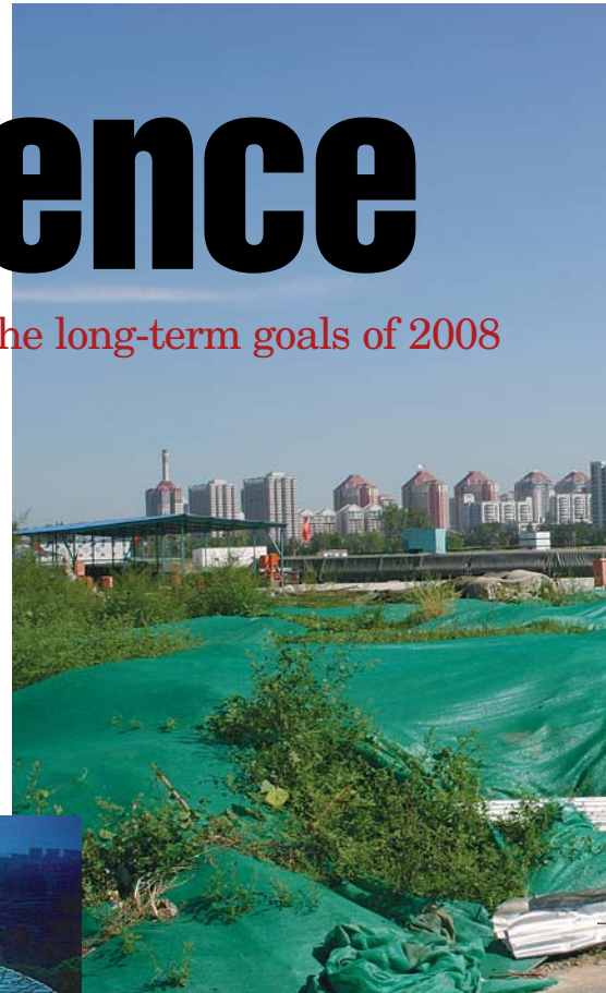
EMPTY NEST: This August 31 photo shows the site of the "Bird's Nest" after construction was halted on July 30
