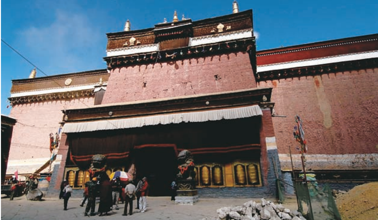
FACELIFT: Saga Monastery is undergoing extensive renovation work. Restoration of Tibet's three major cultural heritage sites, including the Potala Palace, Norbu Lingka and Saga Monastery, is expected to be completed this year
