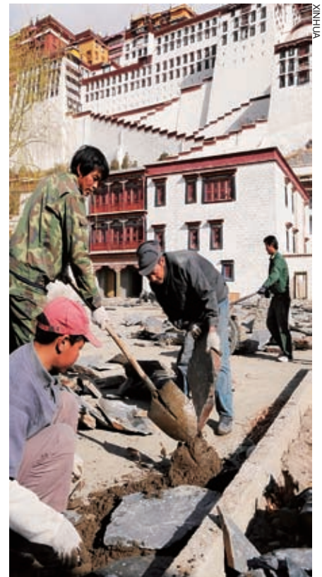
TOUGH JOB: Workers renovate the famous Potala Palace in Lhasa. Renovation work can only be carried out during a short period of the year in Tibet, due to the region's high altitude and freezing winter temperatures
