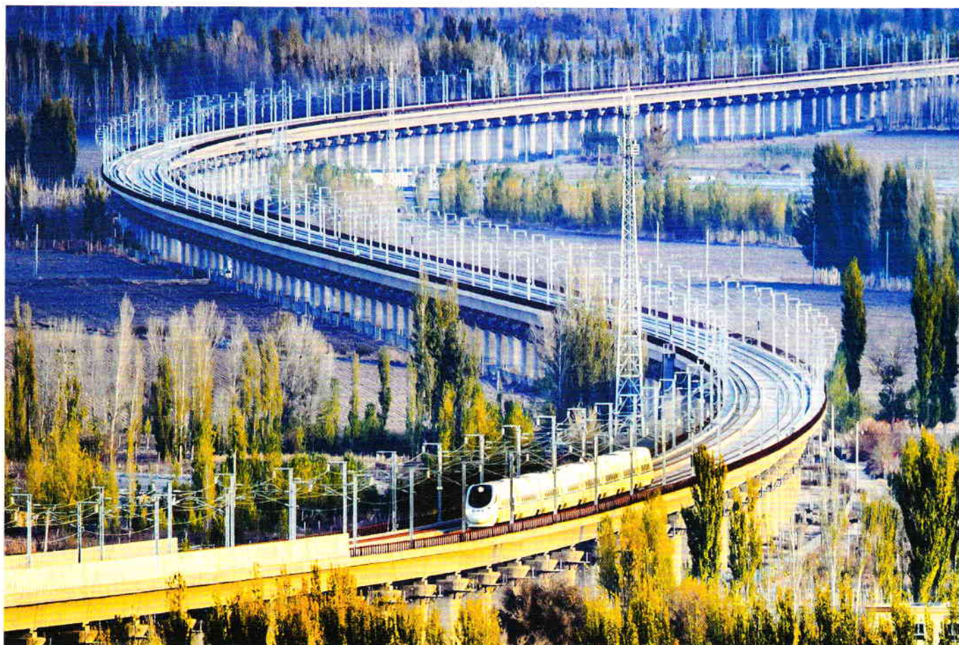
A bullet train runs on a railway bridge in Hami, northwest China's Xinjiang Uygur Autonomous Region
