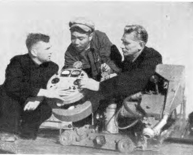
Two Soviet specialists Fyedorov and Mordovsky showing a worker of the Sino-Soviet Shipbuilding Company in Dairen how to operate an automatic welder
