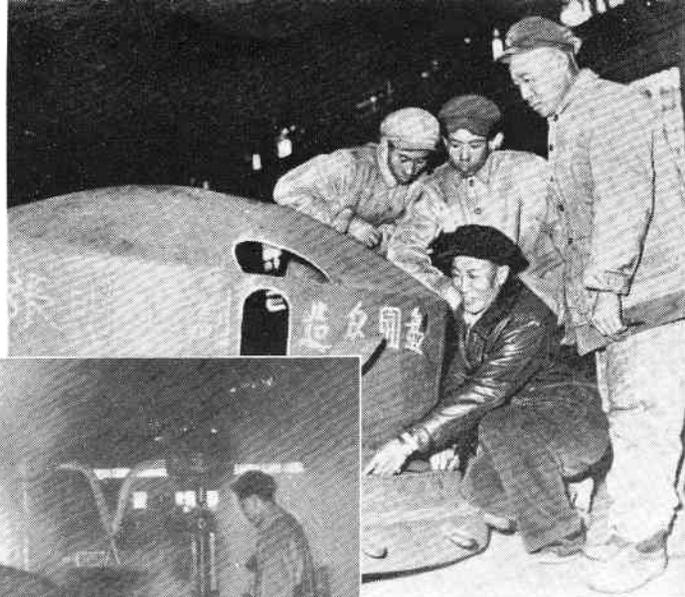
Model worker Chang Ming-shan (*kneeling*) with his invention, the "reverse repeater," which automatizes the most dangerous process in rolling steel bars
